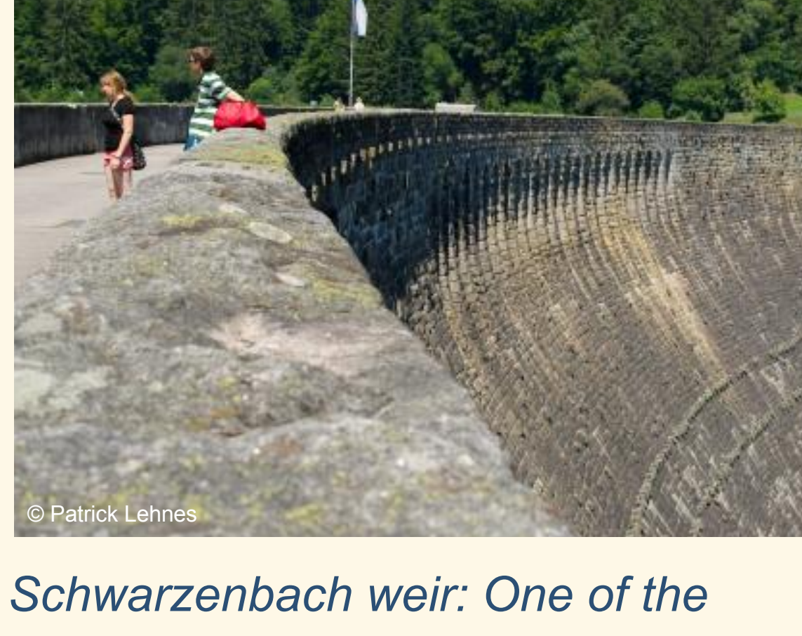
Schwarzenbach weir: One of the oldest pumped-storage power plants in Germany.
